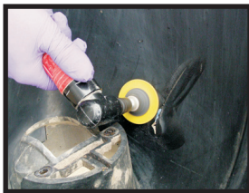
Prepare the damaged area
